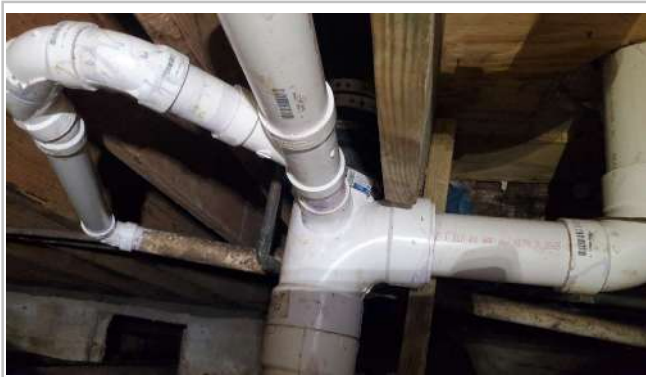
Crawl space PVC pipe view.
